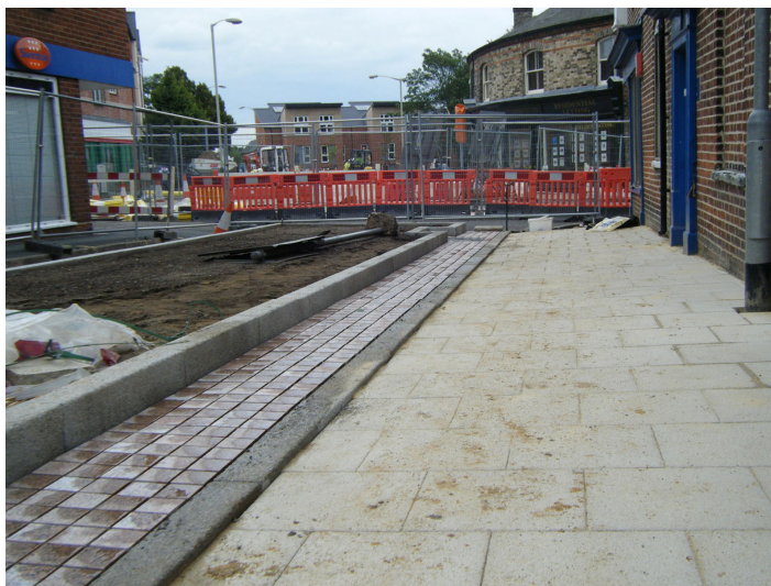
Eastern end of Bakers Road looking towards St Augustine's Street, with the new raised planting bed and paving works well underway.
