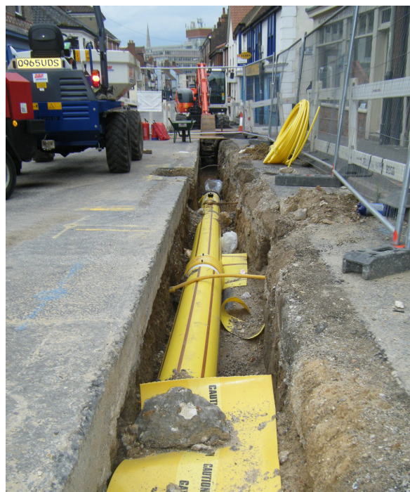
Looking south along St Augustine's Street, showing 12" gas main in trench.
